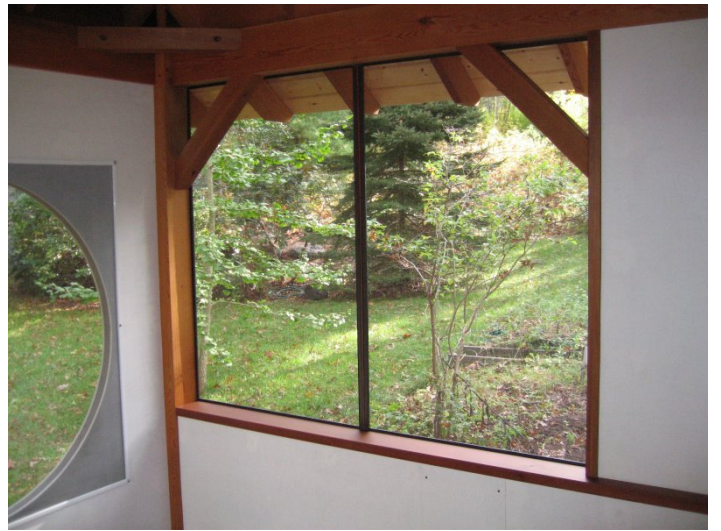
Screens were made from standard hardware-store fiberglass screening and snap-together aluminum frame kits. They were held in place with molding cut from scrap mahogany decking.
