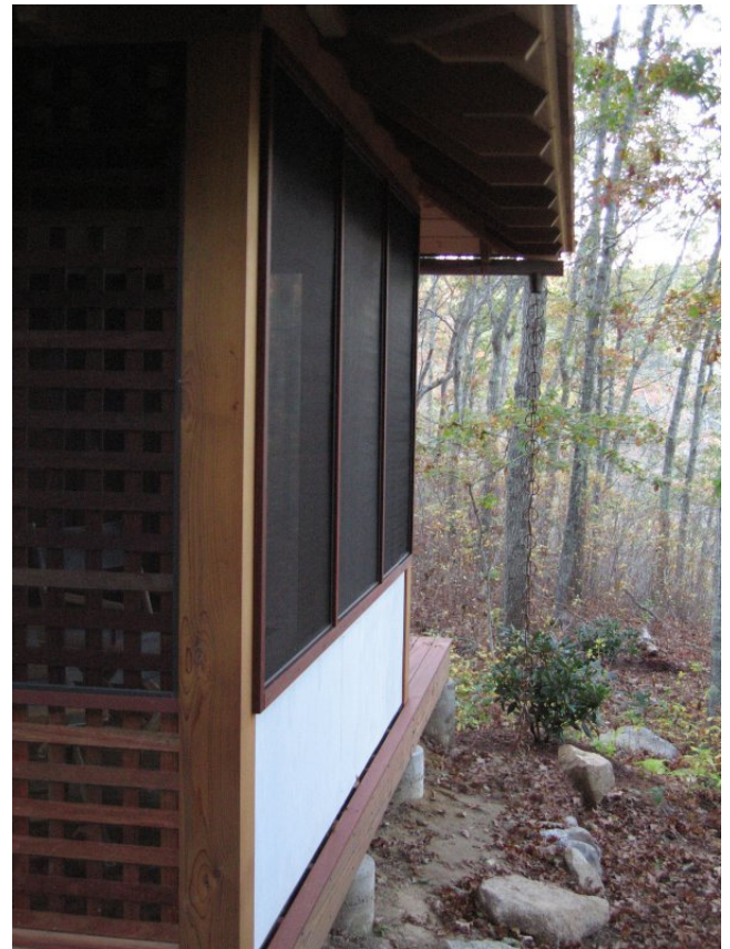
North side – grid window on left has screened top, lucite panel bottom
