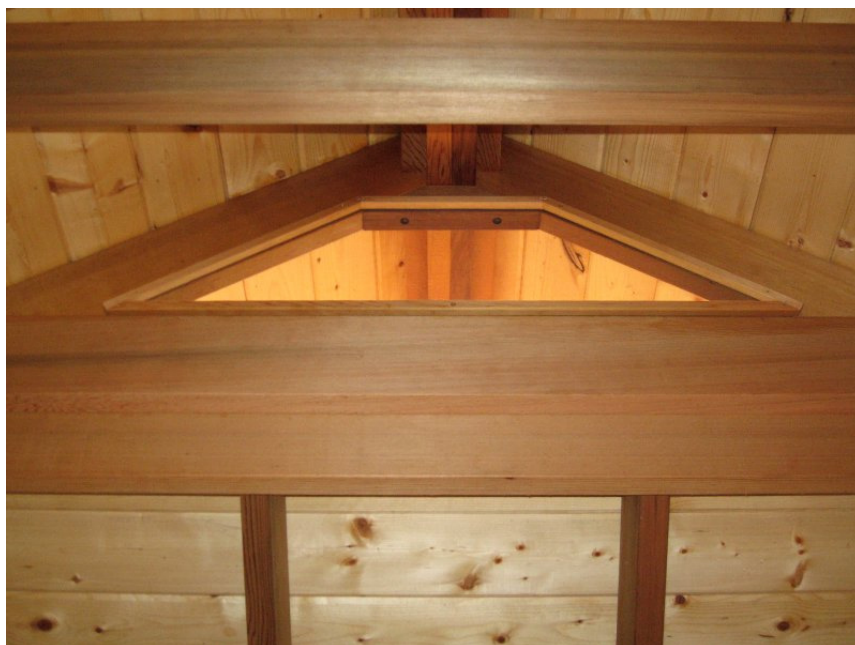
Ridge opening – cedar-framed screen inside
