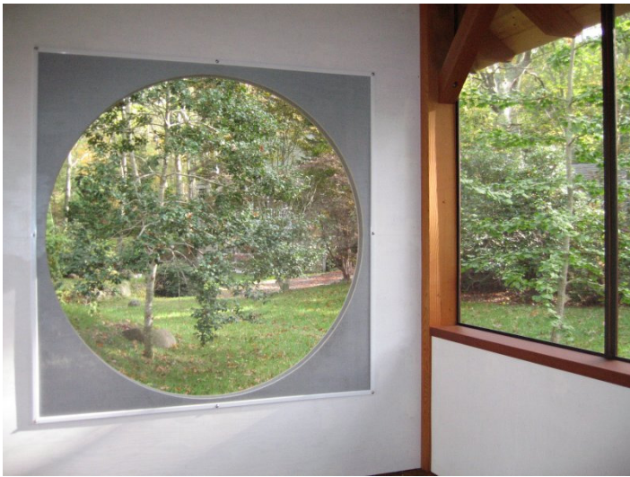
Screens were made from standard hardware-store fiberglass screening and snap-together aluminum frame kits. They were held in place with molding cut from scrap mahogany decking.
